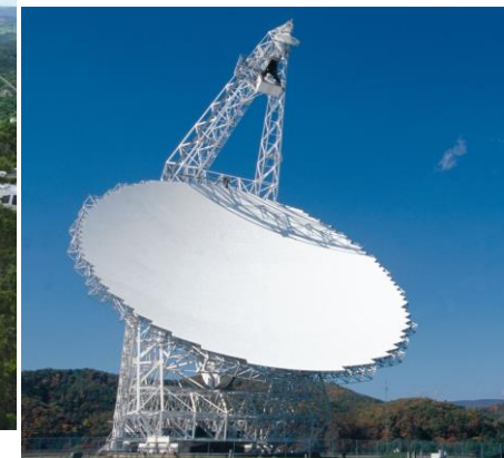
Fig. 6: Green Bank Telescope, world's largest fully steerable radio telescope. [NRAO/AUI/NSF]
